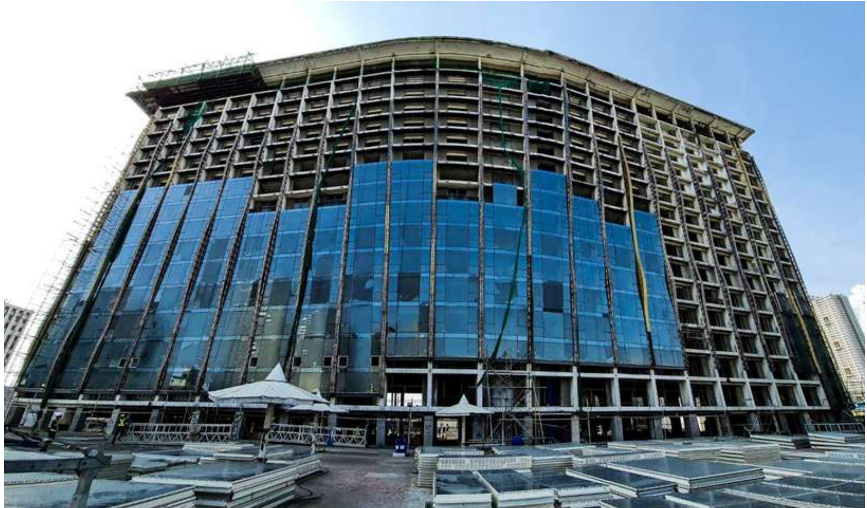
Installation of curtain walls and fins
