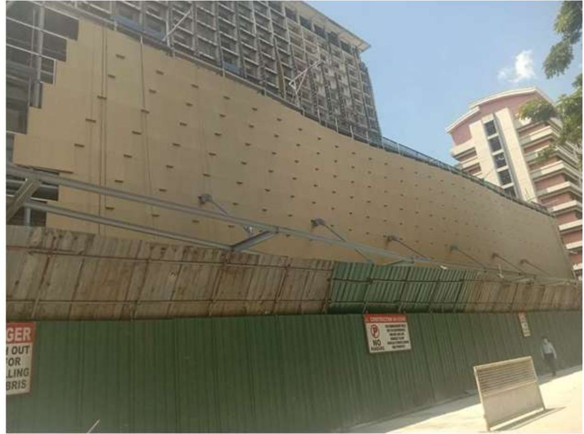
Installation of aluminum composite panels
