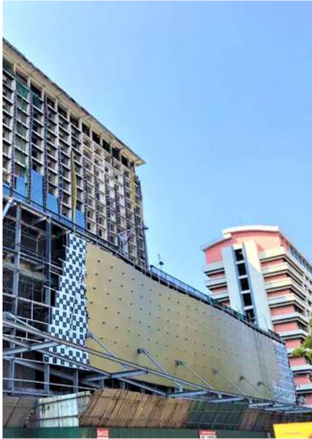
Installation of aluminum composite panels
