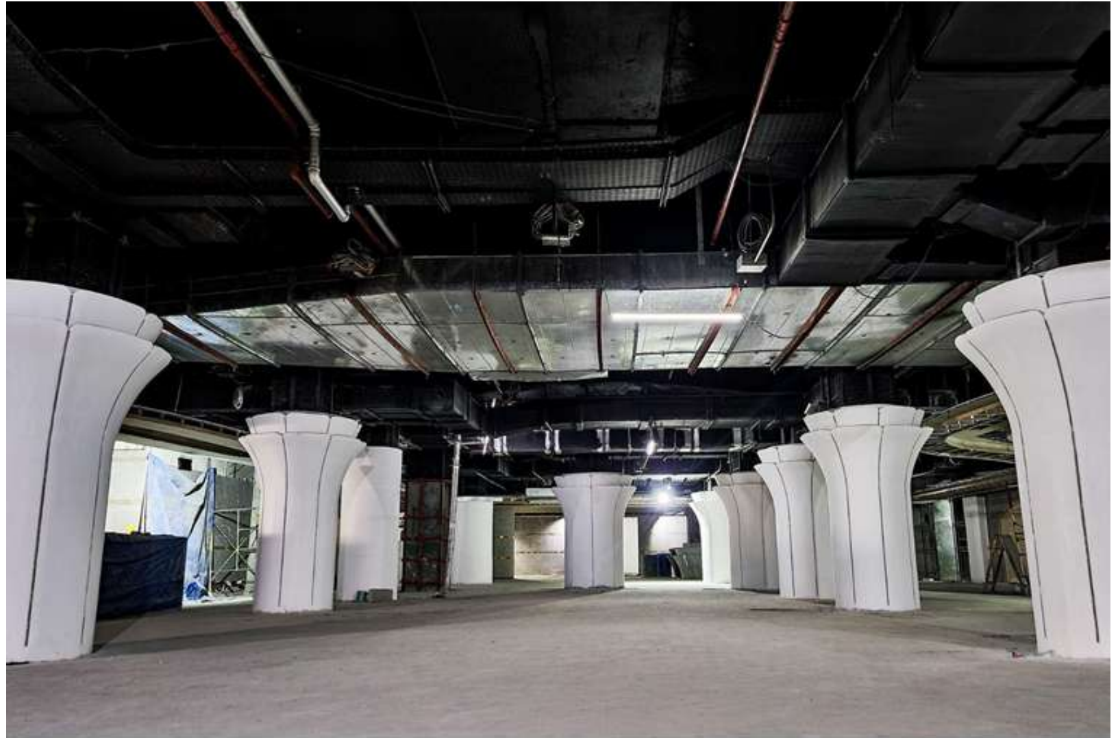
Installation of GFRC column cladding
