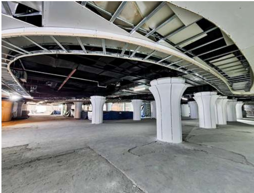
Installation of ceiling boards
