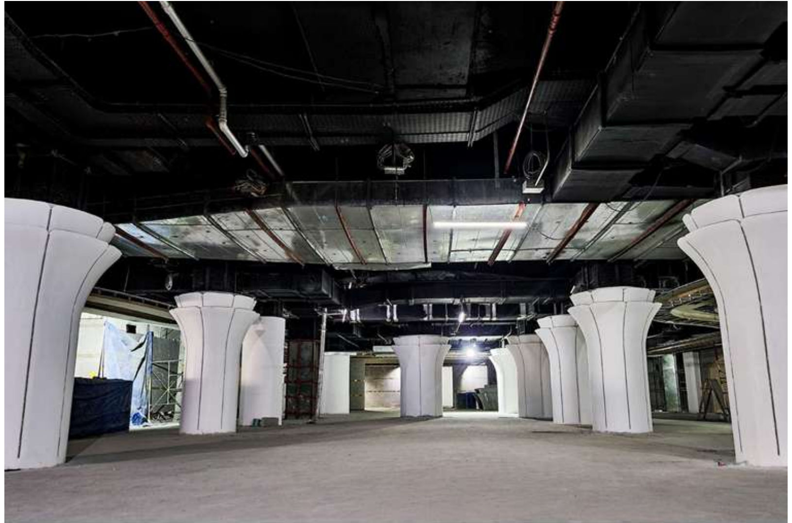
Installation of GFRC column cladding
