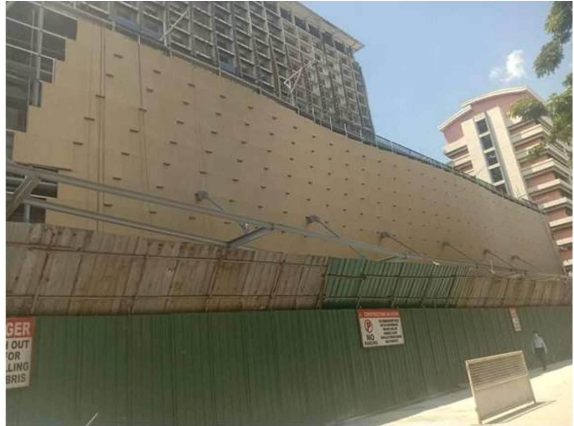
Installation of aluminum composite panels
