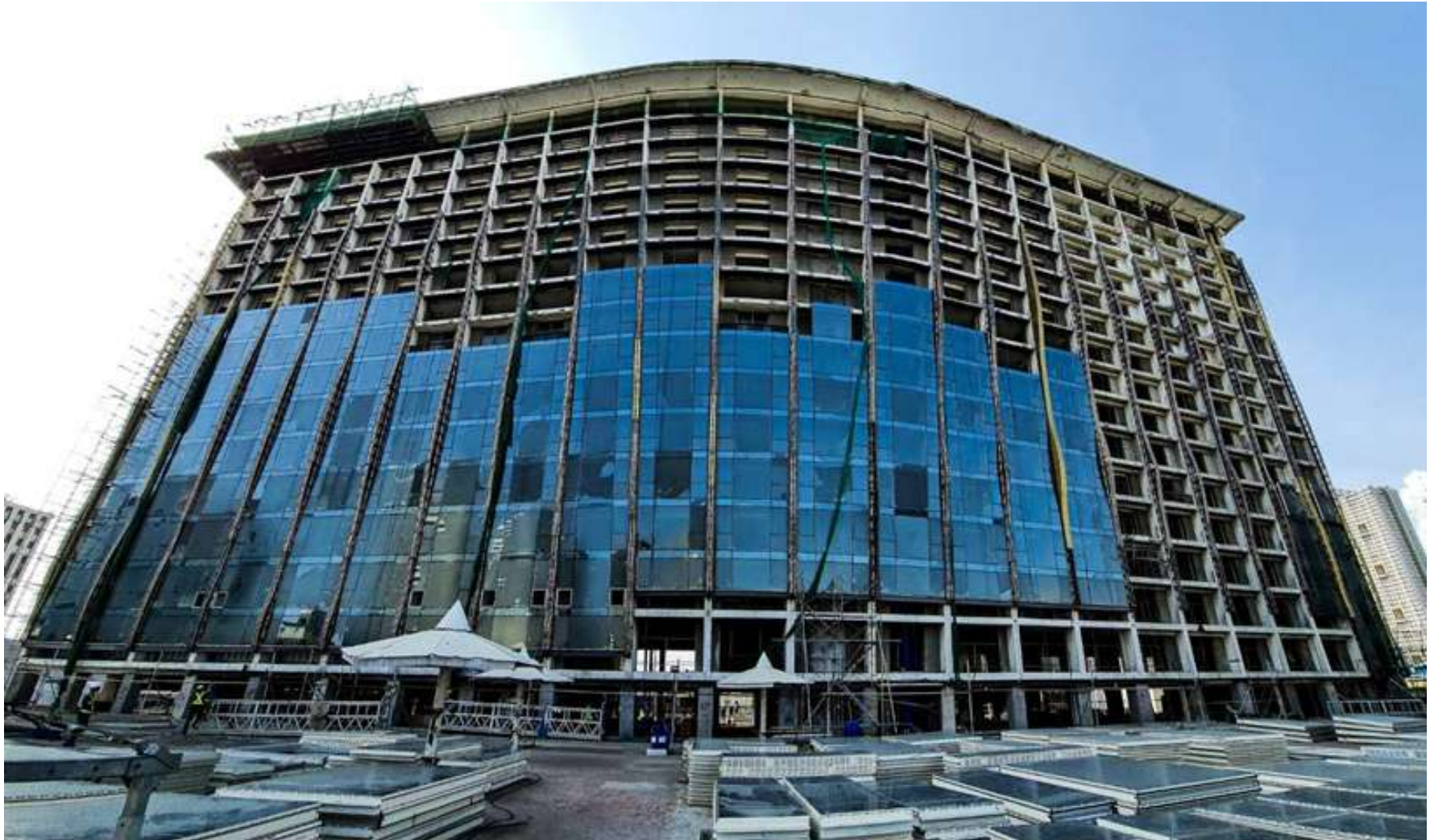
Installation of curtain walls and fins
