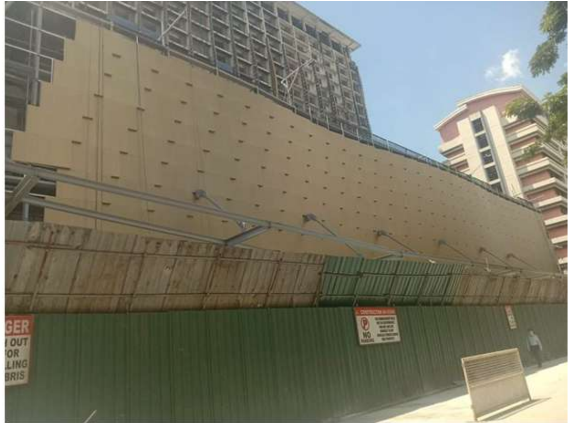
Installation of aluminum composite panels
