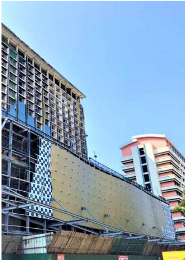
Installation of aluminum composite panels
