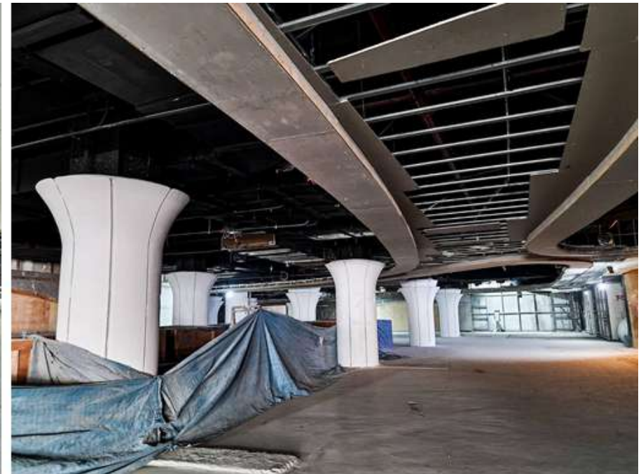
Installation of ceiling boards
