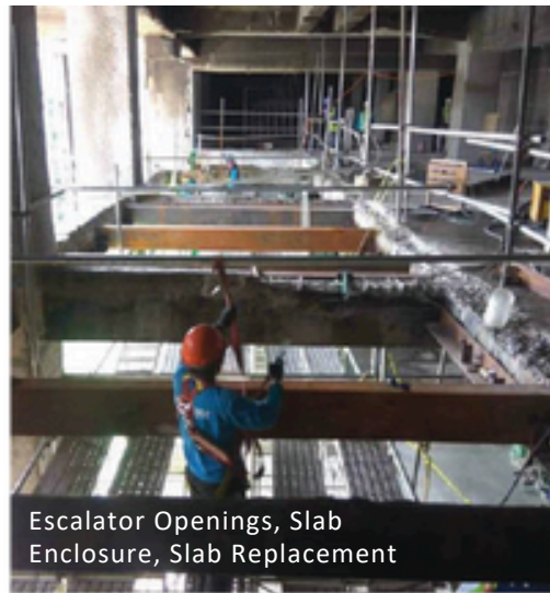
Escalator Openings, Slab Enclosure, Slab Replacement
