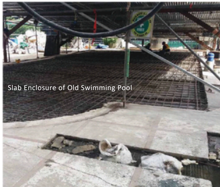
Escalator Openings, Slab Enclosure, Slab Replacement
