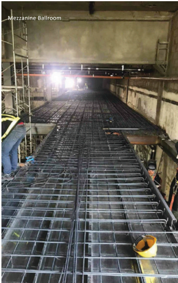
Escalator Openings, Slab Enclosure, Slab Replacement
