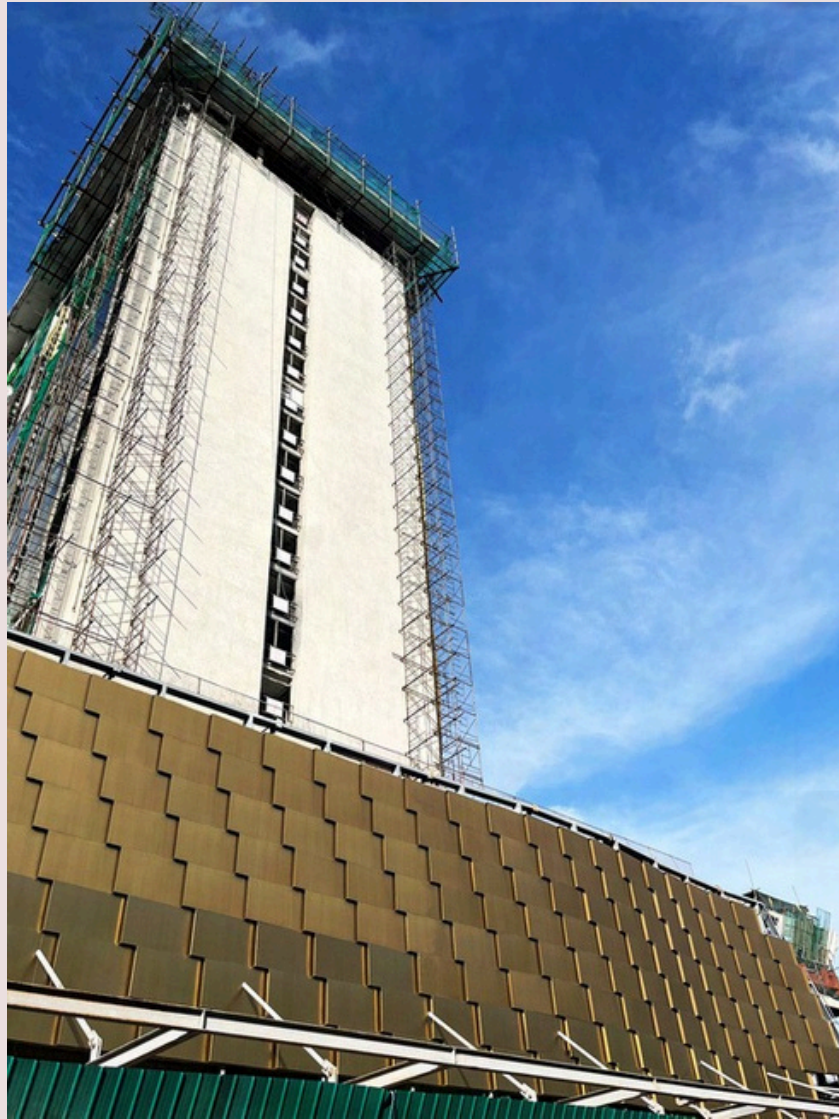
INSTALLATION OF ALUMINUM COMPOSITE PANELS
