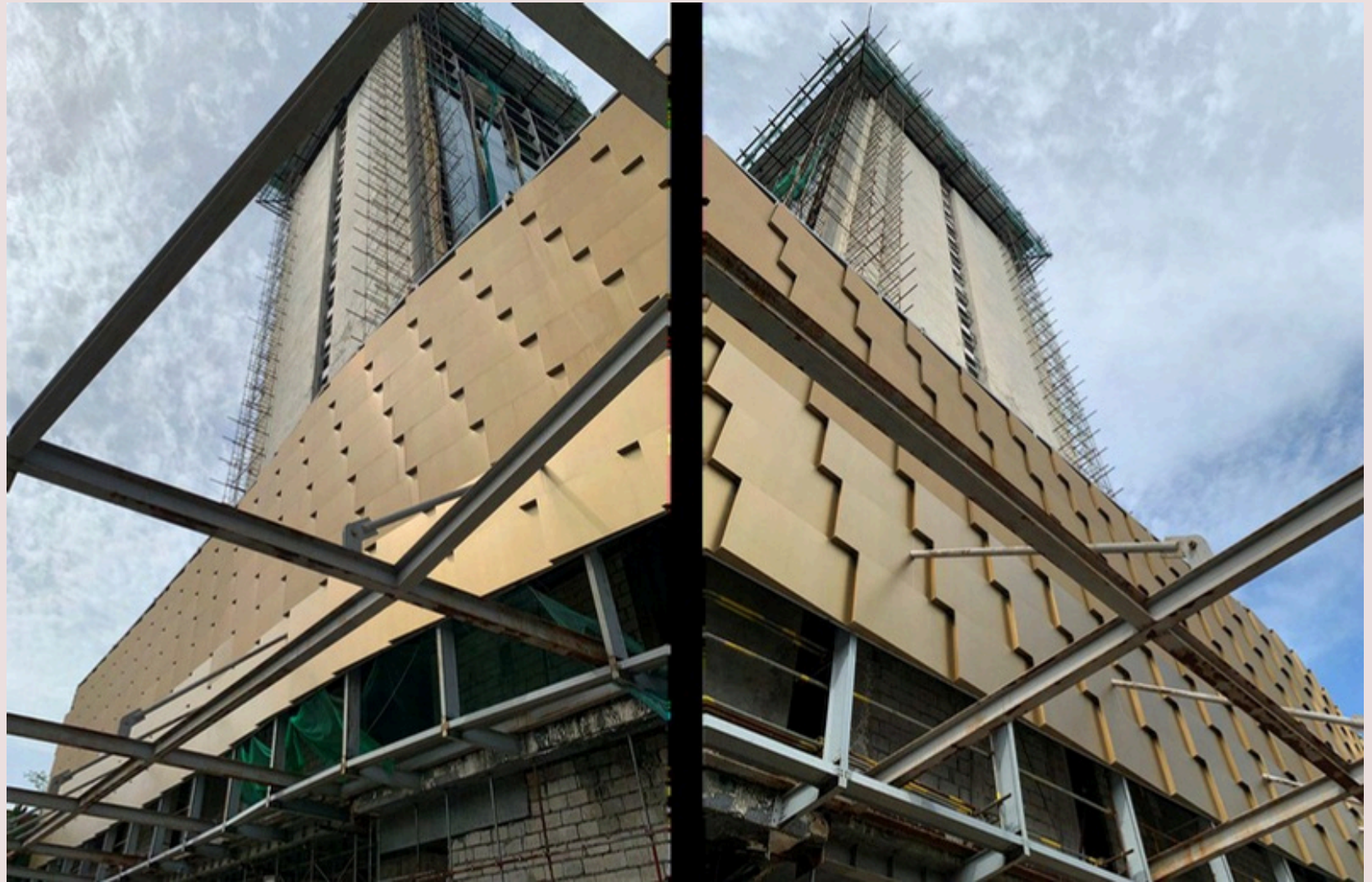
INSTALLATION OF ALUMINUM COMPOSITE PANELS
