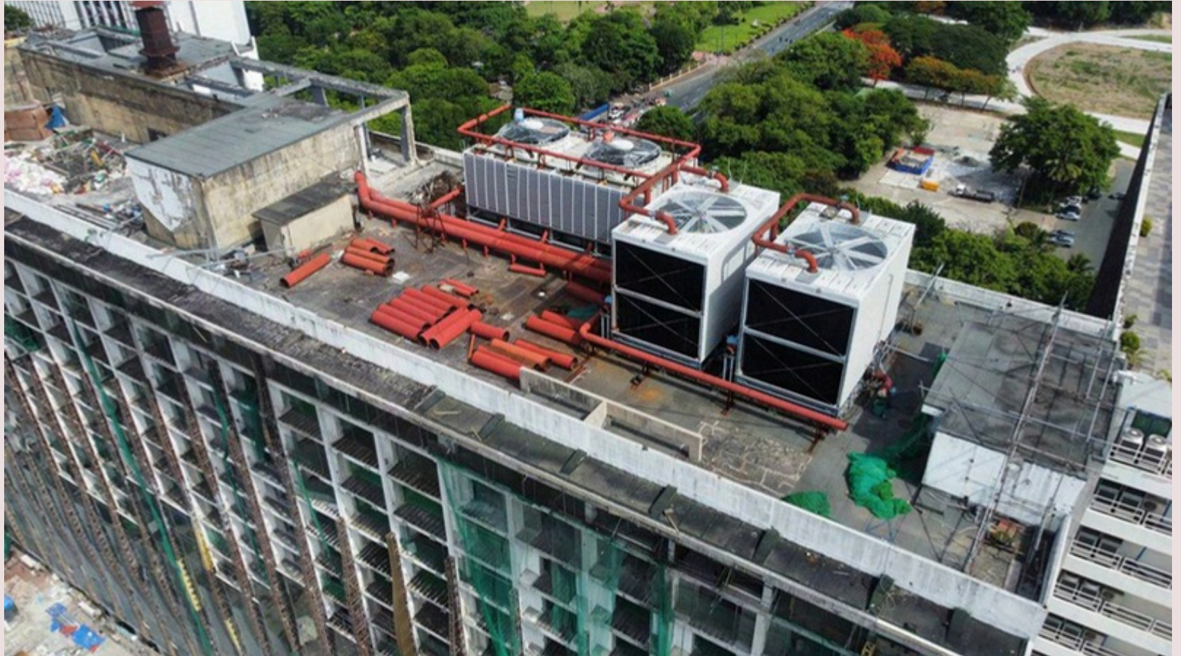
COOLING TOWER PIPING WORKS
