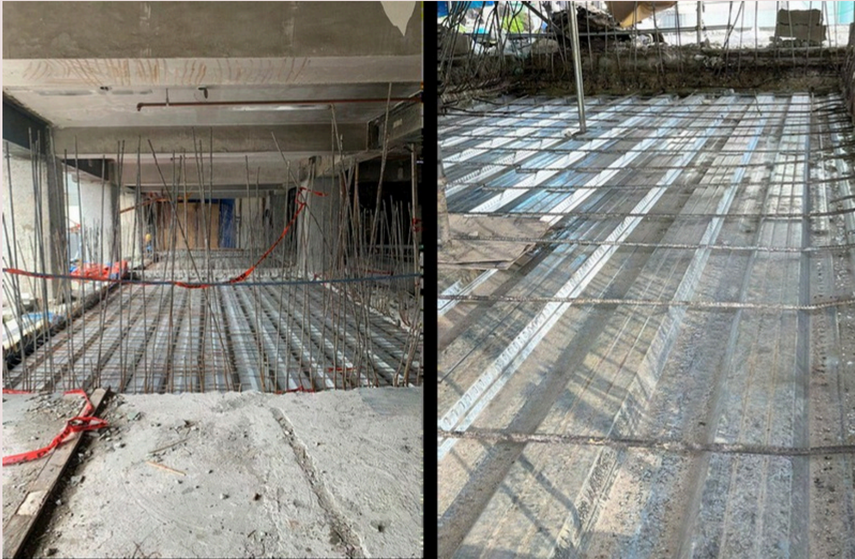
ONGOING REPLACEMENT OF SLAB
